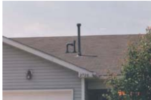
Figure 47 Example of a 1990s house sample with roofing rated as adequate.
