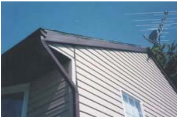
Figure 36 Example of aluminum fascia covering older fascia material on a 1970s sample house (rated good by inspector).
