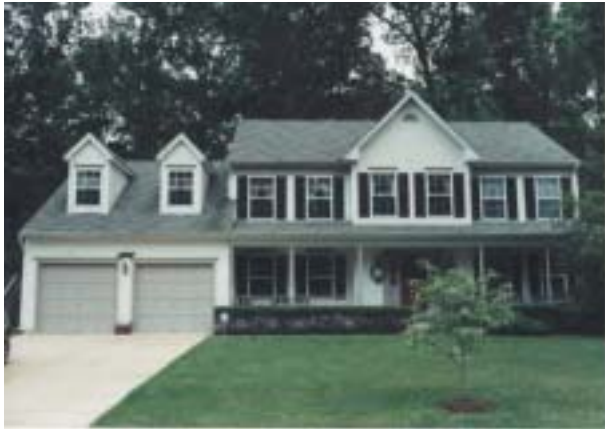
Figure 22 Example of good rating for site grade and drainage.
